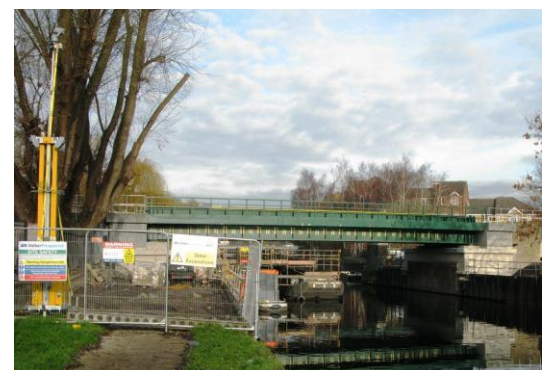
A new Bridge 32 was installed over the Lea Navigation during the New Year holiday. It is still awaiting the electric wires on 2 nd February 2017.
