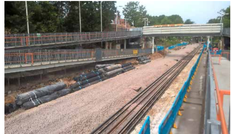
▲ Looking north-east in the direction of Blackhorse Road station and the Gospel Oak end of the line, work continues to lengthen the platforms at Walthamstow Queens Road to accommodate four-car EMUs once electrification is complete. PAUL STEPHEN.
