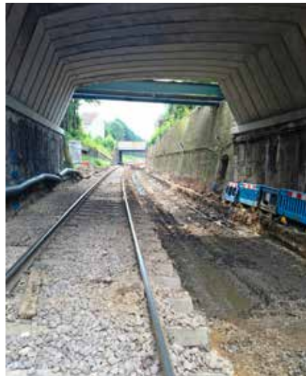
▲ Track lowering at the south end of Walthamstow Queens Road station. The Up line trackbed has been excavated to a depth of 50cm below the height of the adjacent Down line. Queens Road bridge - one of the lowest on the line - is in the background. NETWORK RAIL.
