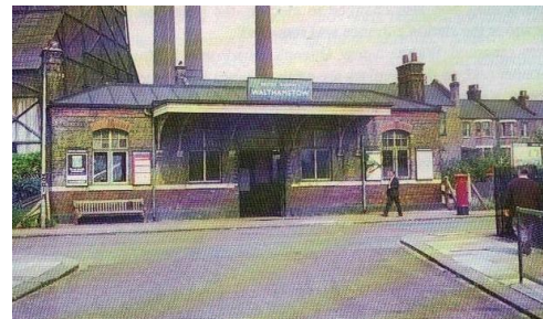
Seen in early 1968, the station was renamed Walthamstow Queen’s Road on 6 th June that year. The chimneys & cooling towers of Walthamstow Power Station can be seen behind the station. [Photo: J. E. Connor]
